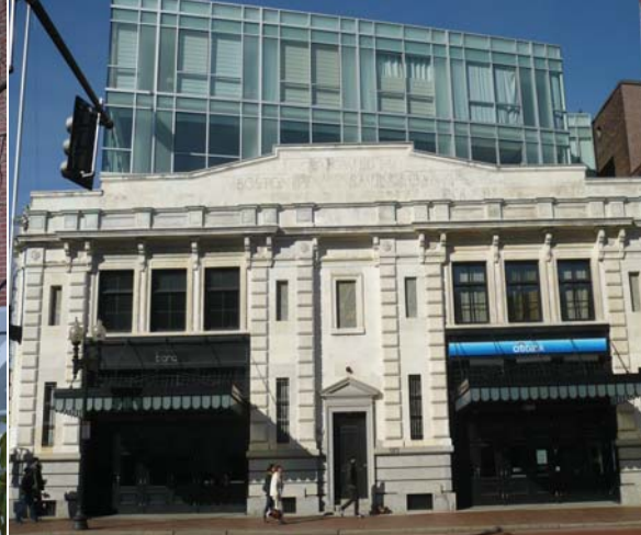
The marble and granite building constructed in the Renaissance Revival style between 1911 and 1917 and renewed with the help of South End Historical Landmarks and the Boston Redevelopment Authority. The renovated building - featuring three new floors of glass set back from the existing building - hosts the South End branch of CityBank, which also comes with a $75,000 pledge over a three-year period to support the Washington Gateway Main Street Program.
